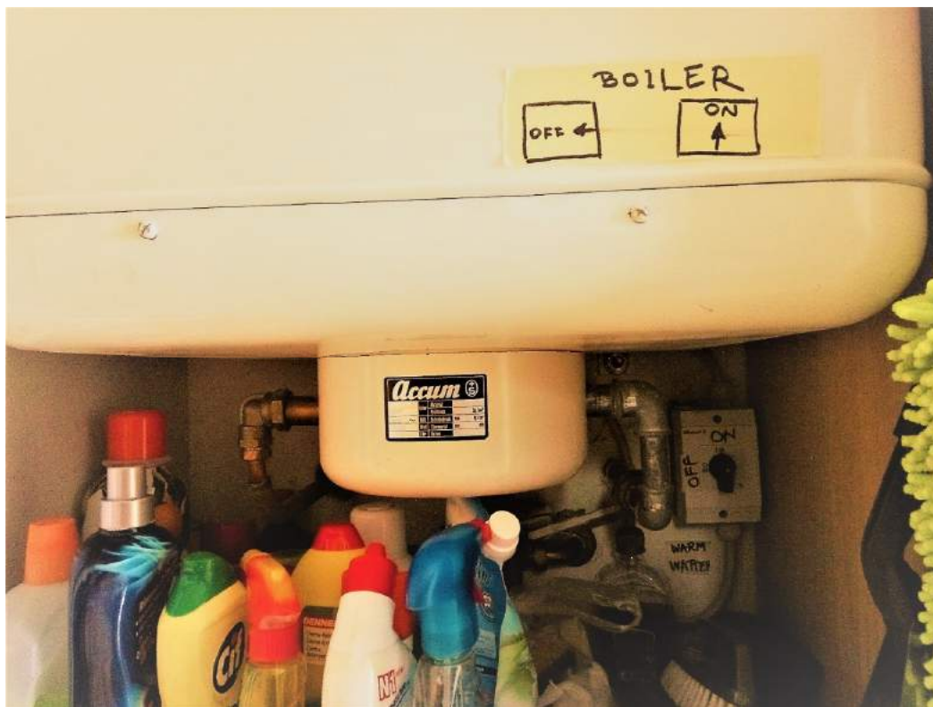
Figure 50 - Boiler switch
